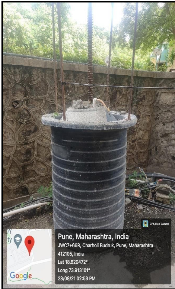
Biogas Plant Located at Behind Canteen Area
