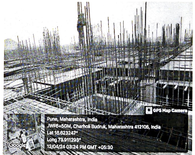
Reinforcement of lift, beam and column
