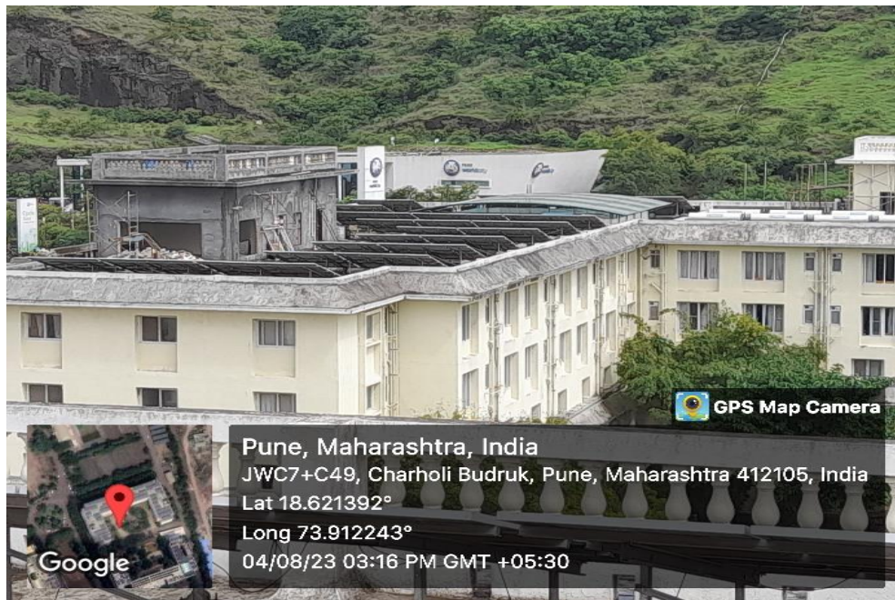
Solar Panel located on Roof of Hostel Building
