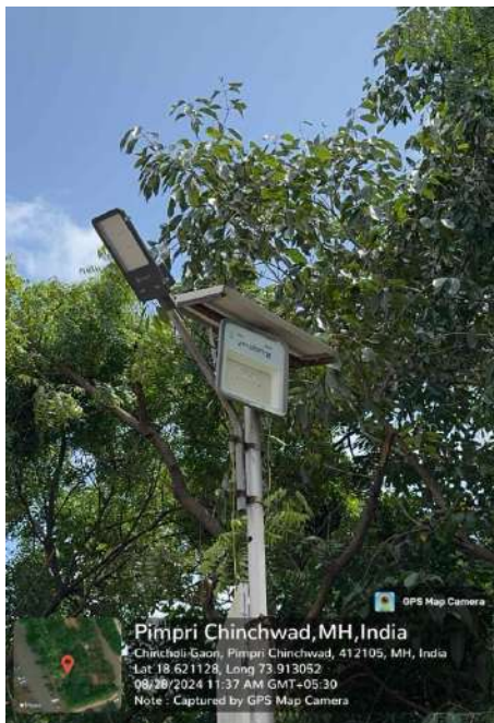
Fig1: Solar charged outdoor LED lights
